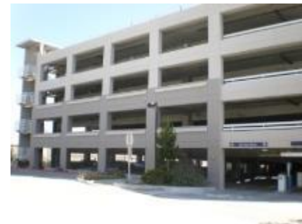
Structured Parking Garage
