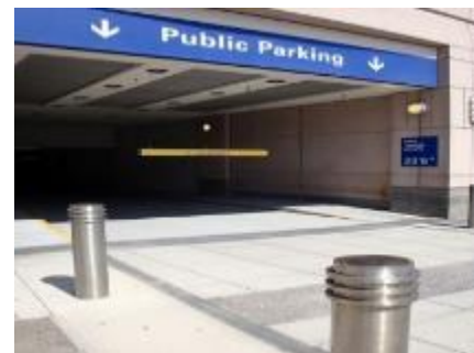
Subterranean Parking Garage
